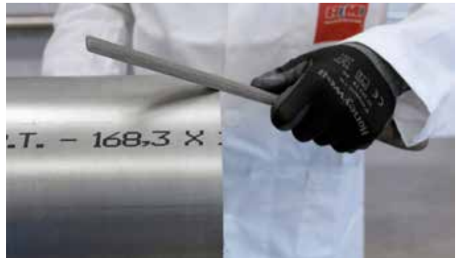
Figure 13 - Deburring the pipe
