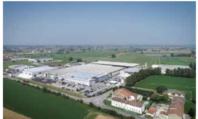
Figure 1 – Campitello head office and factory
